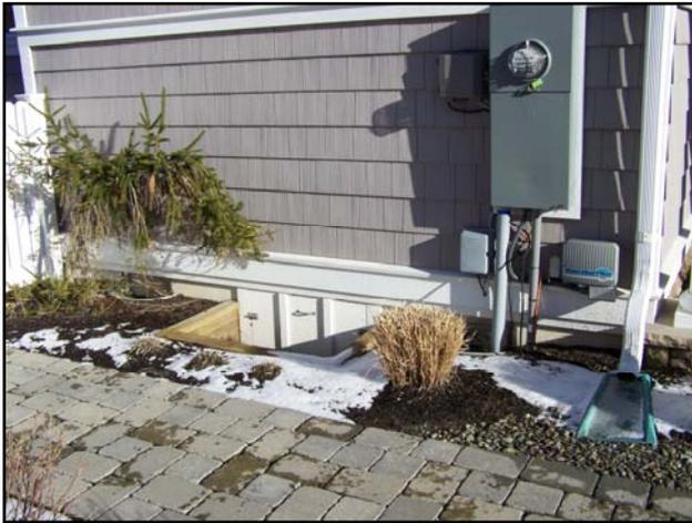
Photo 1: Flood vent & crawl space below grade
