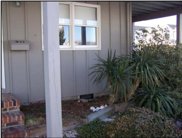
Photo 2: Flood vent & non-conforming crawl space
